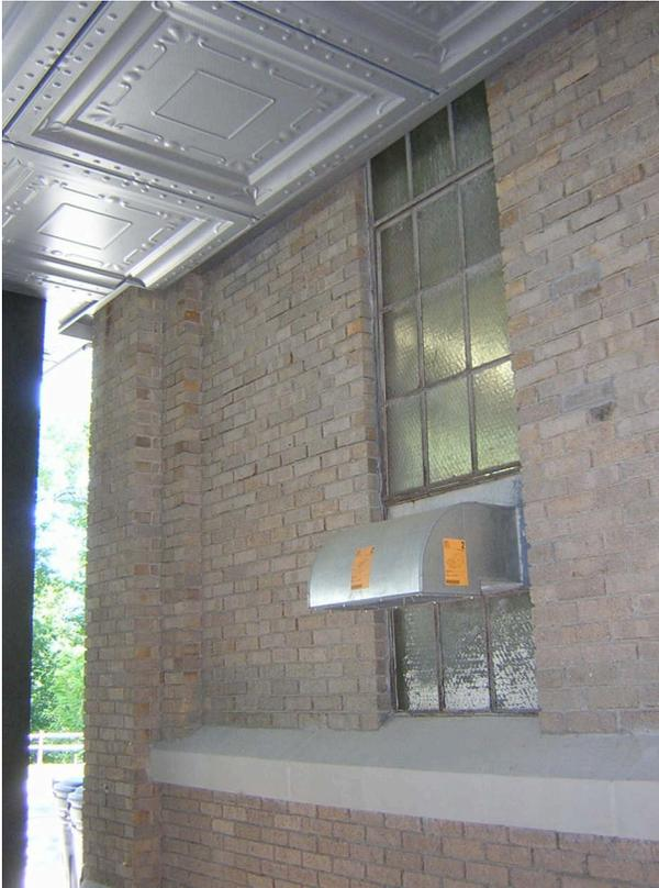
**Figure 3.** Lack of opening protectives in fire barrier between Rand and Milstein Hall (photo by J. Ochshorn, June 2013)
